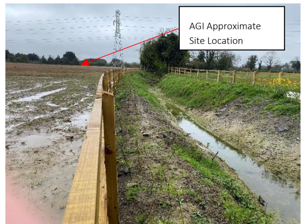
Eastern Drainage Ditch – South East Corner of Site (Camera Facing North)
