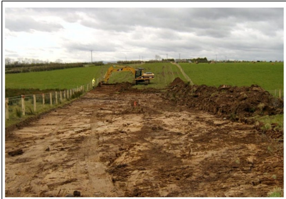
Figure 2-13: Image of Topsoil Removal within Working Width
